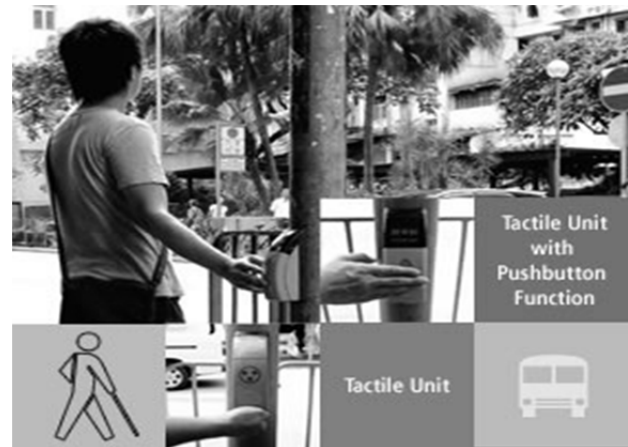
Fig. 14: Electronic audible traffic signal system
